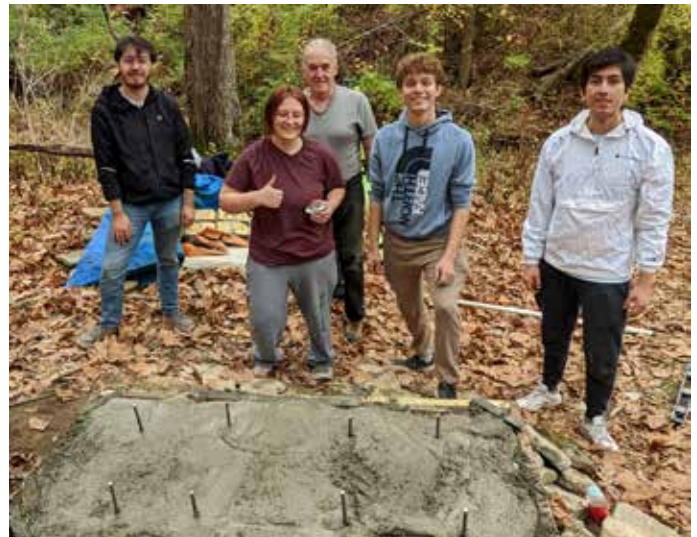
Finished the footing for the Bridge
